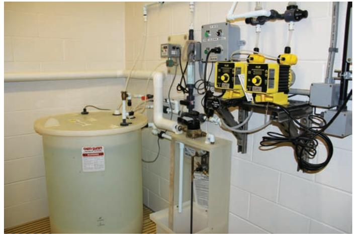
**The fluoride saturator and associated pumping equipment is checked daily to ensure proper operation. Operators also test the fluoride level and make adjustments as needed during these daily inspections.**
