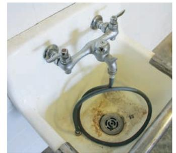
**A hose left in a sink or basin is an example of a common cross connection in a home. Fortunately, this faucet has a vacuum breaker air valve installed to prevent a back flow from occurring.**
