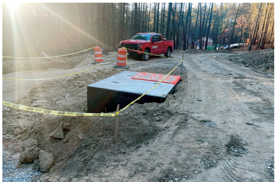
Foundation and piping work is underway in South Acton (left) while the meter vault for the bedrock wells in Acton Center (right) awaits electrical and piping connections to be made.
